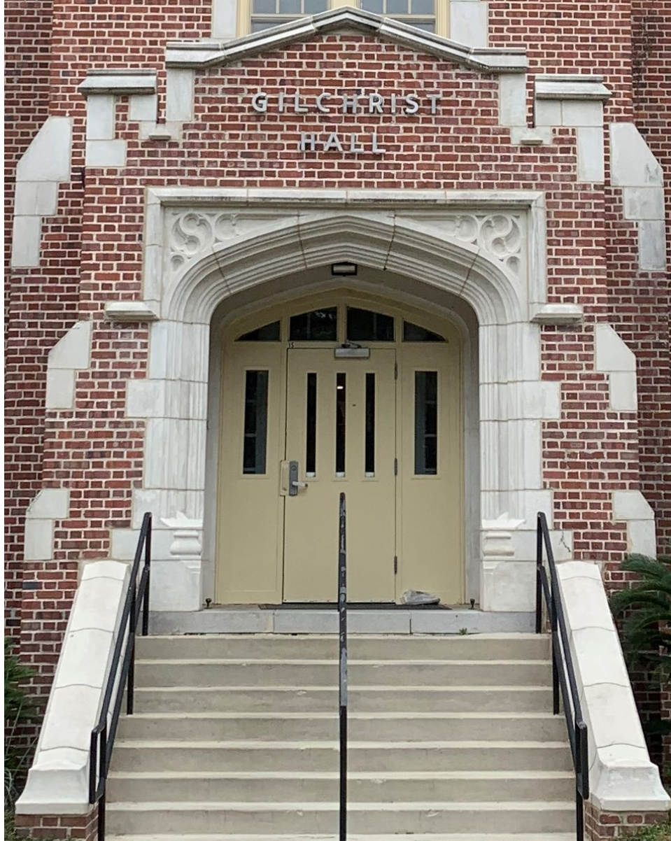
Photo 15.4 Jacobean Revival Arch (Gilchrist Hall – 1925)
