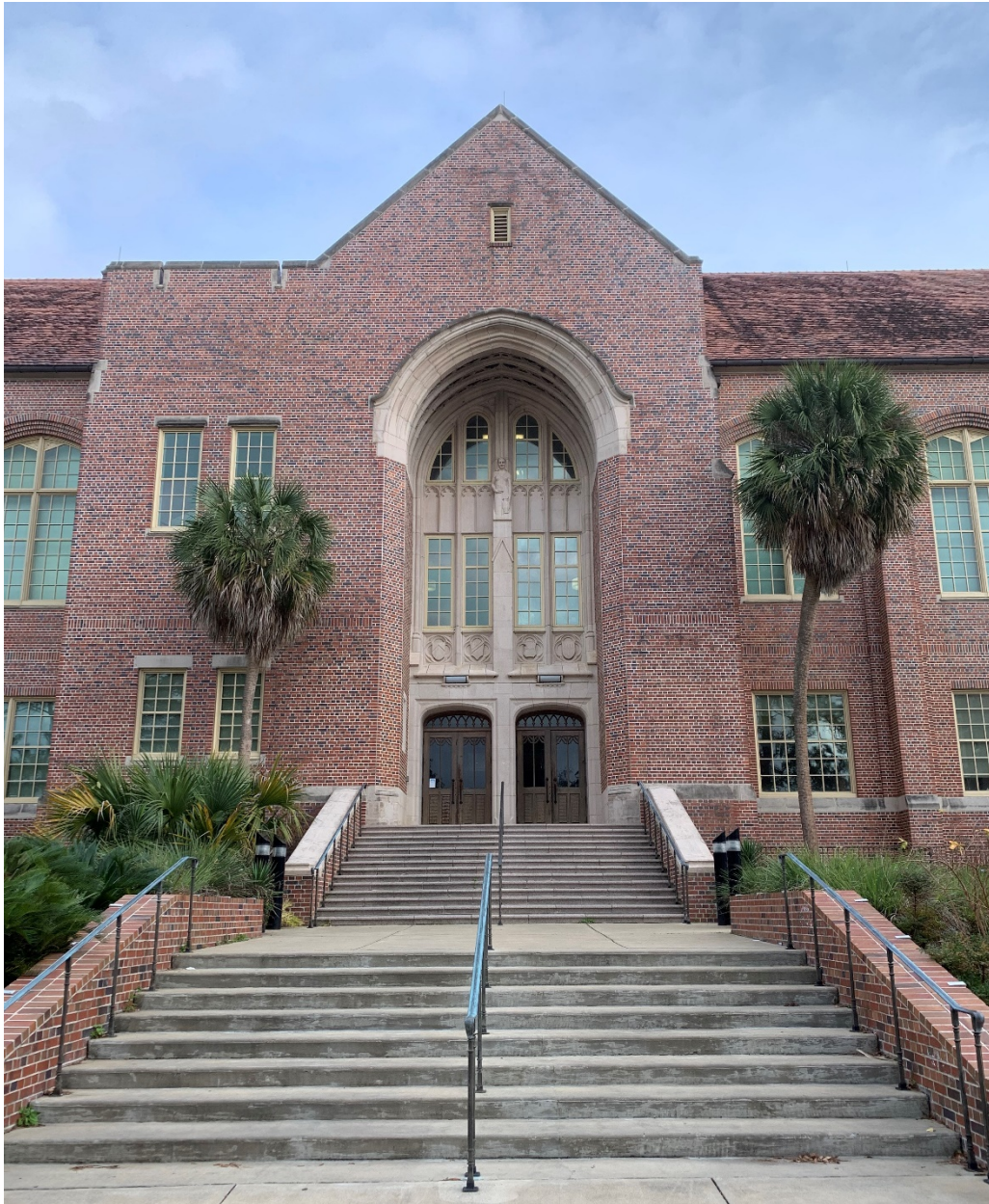
Photo 15.15 Building Raised on Small Podium (Johnston Building – 1913)
